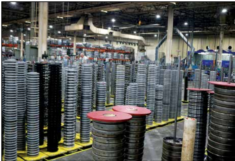
Stacked and ready for the assembly line, completely rebuilt and inspected stators.
